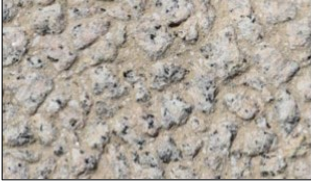
Close-up photograph of the Sculpture Garden aggregate concrete walls.
