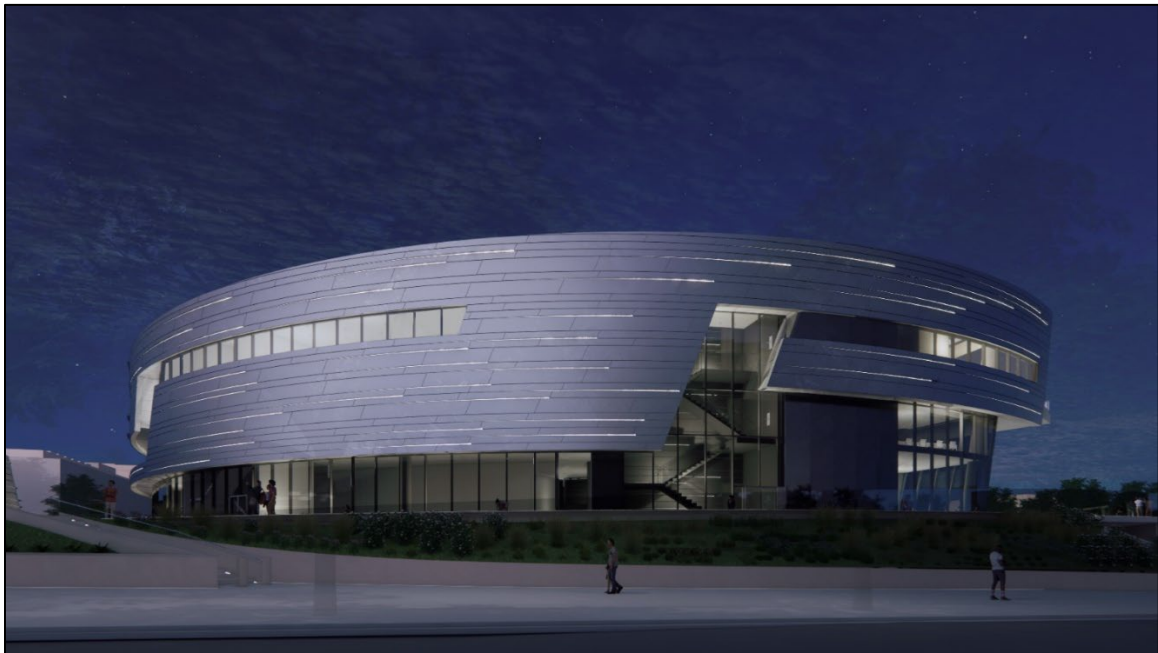
East elevation rendering at night of BLC and Hass Observatory with the integrated façade lighting within the metal panels. (Perkins&Will, 2024)
