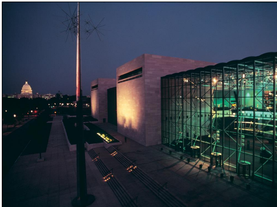
Original Curtain Wall Glazing, 1976.
