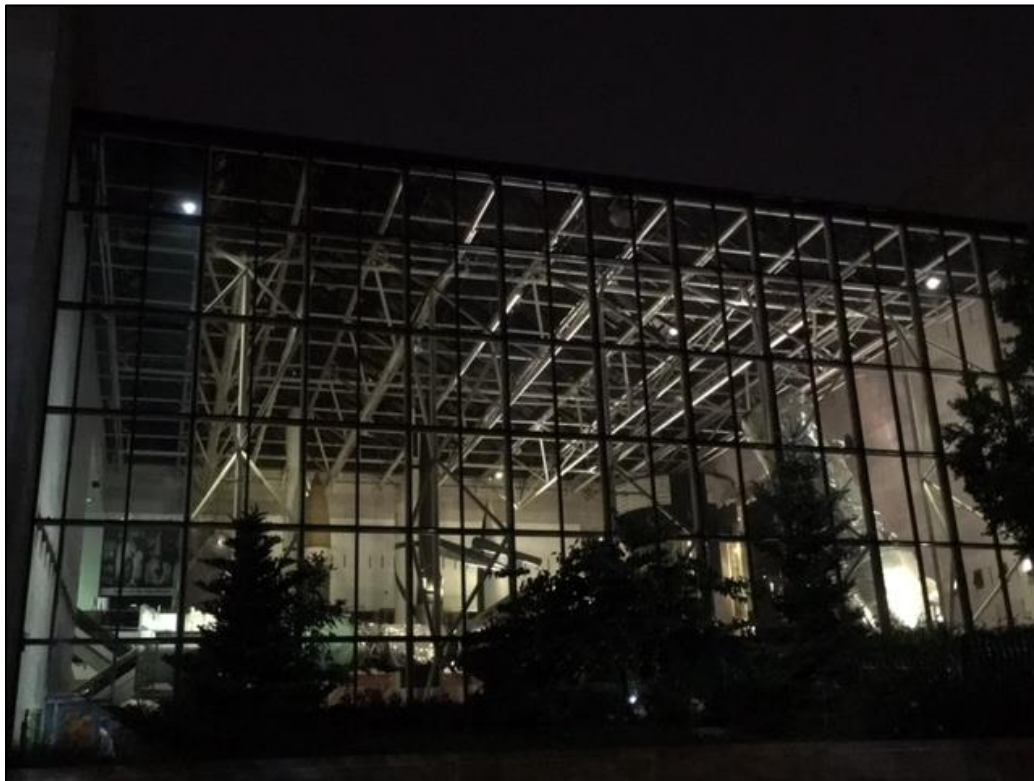
View of Atrium at Night, Glazing Mock-up at Far Left Bays, 2017.
