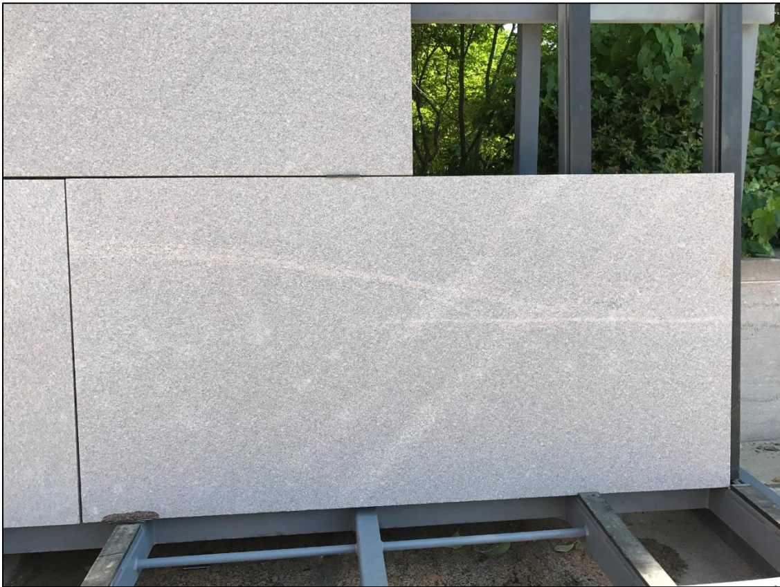
Colonial Rose Granite Mock-up, Sandblast Finish, June 2017.
