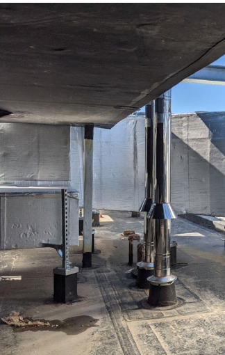
HVAC EQUIPMENT ON OPEN ROOF STRUCTURE REQUIRE OVERHEAD STRUCTURE TO SUPPORT DUCTWORK AND PIPING
