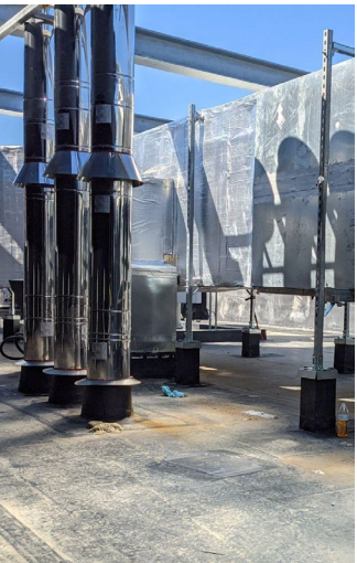
HVAC EQUIPMENT ON OPEN ROOF STRUCTURE REQUIRE OVERHEAD STRUCTURE TO SUPPORT DUCTWORK AND PIPING
