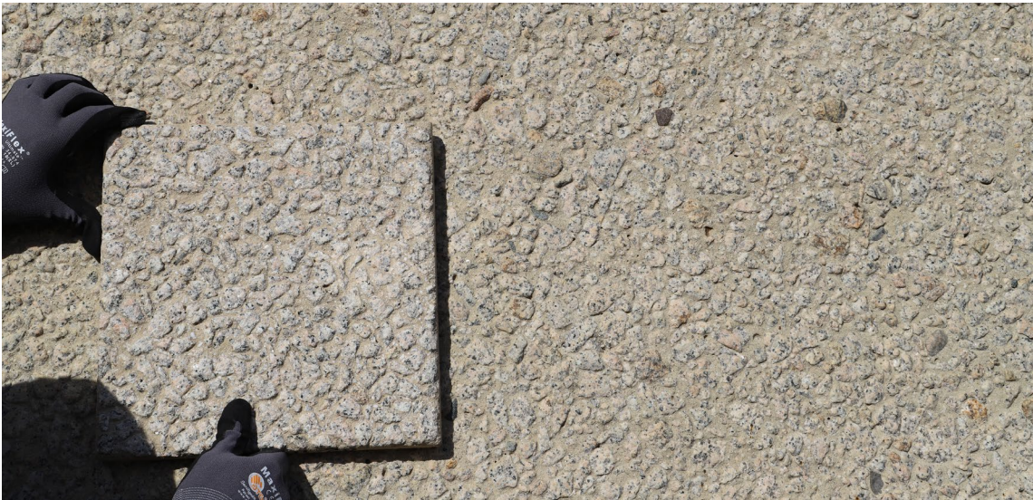
Sample of replacement aggregate concrete held against a historic precast panel, 2019.
