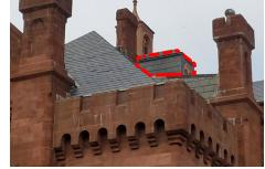
Southeast roof. Existing elevator penthouse to be removed (shown in dashed red lines).
