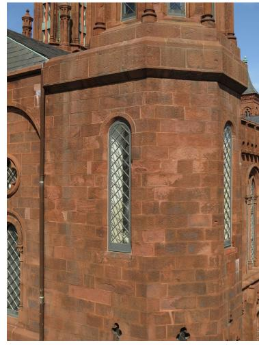
Example of Masonry Spalling & Detachment
