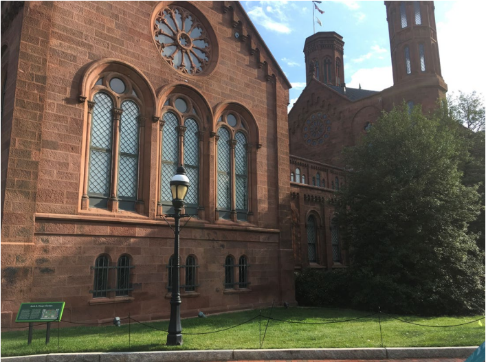
Existing South Facade
