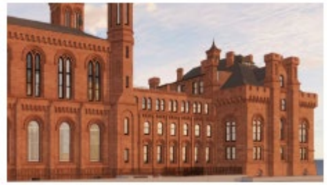
Southeast roof from Haupt Garden. New rooftop penthouse required for elevator overrun.
