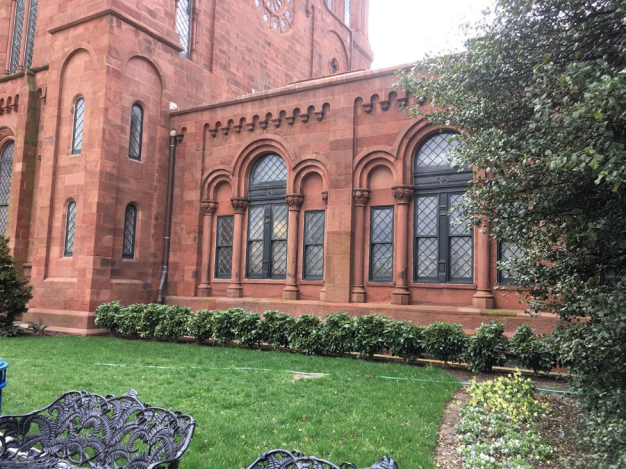
Existing West Range
