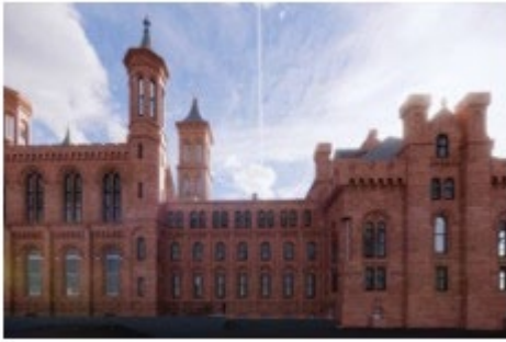
Southeast roof from Haupt Garden. New rooftop penthouse required for elevator overrun.
