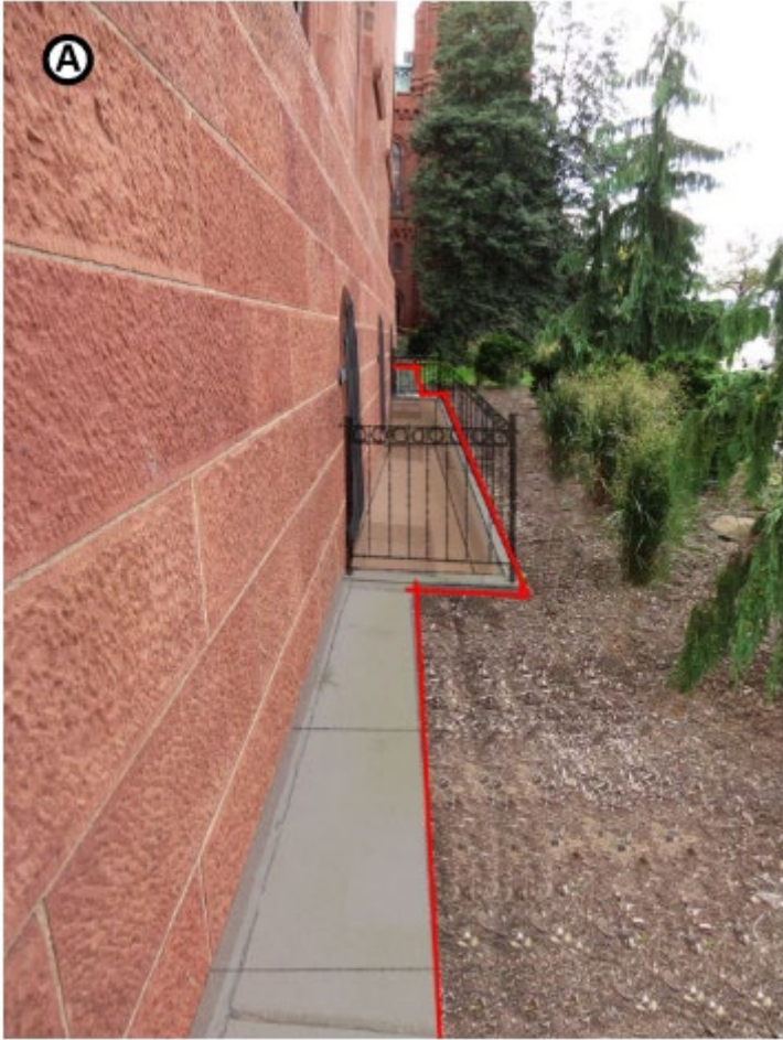
Conceptual Seismic Moat Cover Visualization Note: The design of the railing at the light well is in development- this image utilizes the design of the existing railings at the north entrance ramp
