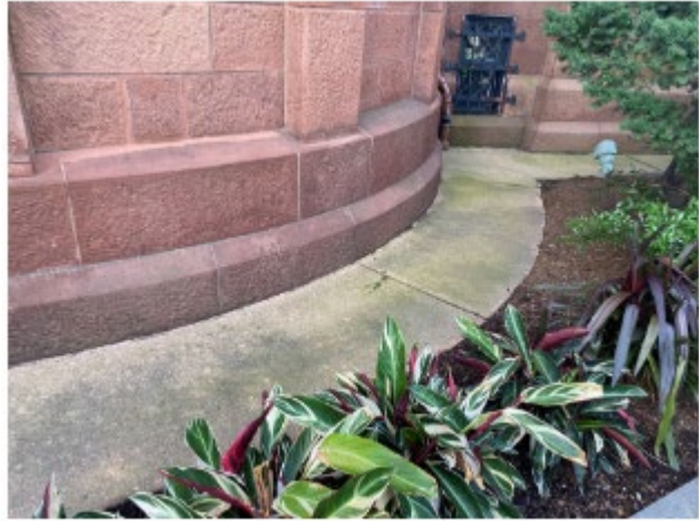
Existing Concrete Apron
