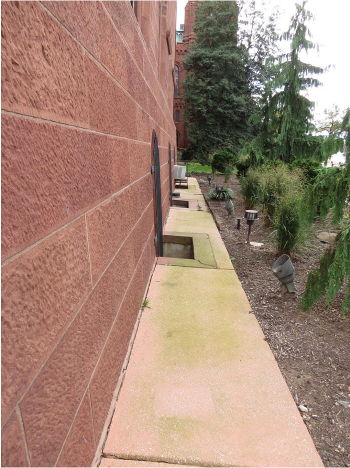
Existing Concrete Apron
