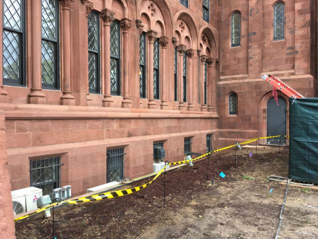
Existing Window Well
