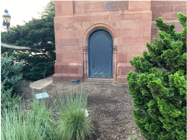
Existing Concrete Apron
