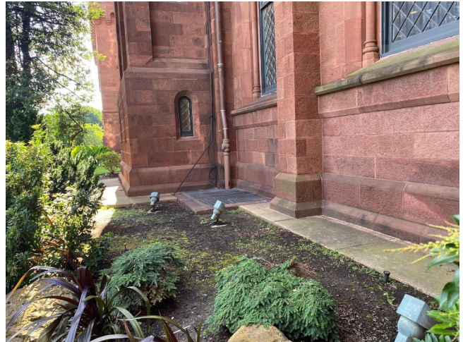
Existing Concrete Apron
