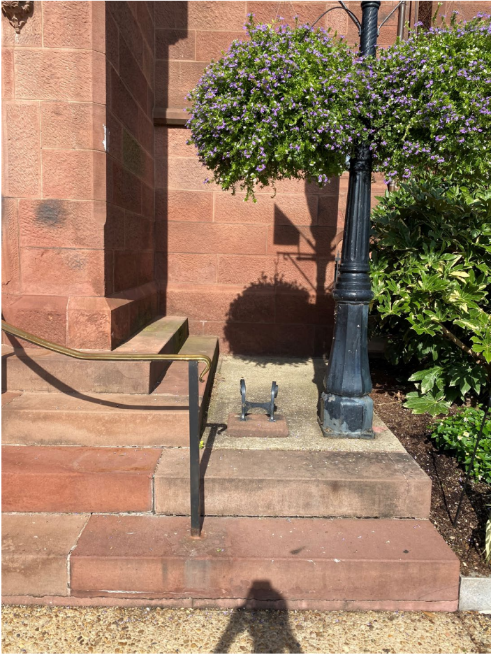
Existing Concrete Apron
