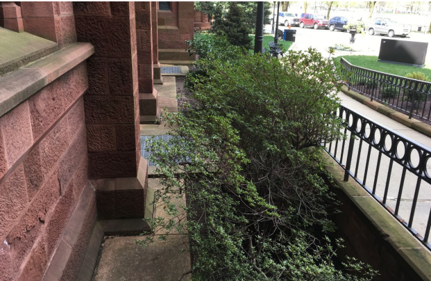
Existing North Tower Ramp
