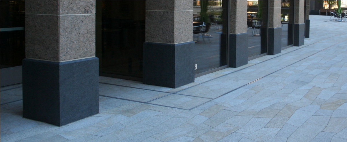
Example showing the joint can be integrated into paver system adjacent to building
