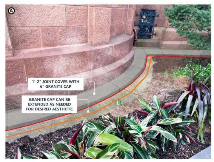
Conceptual Seismic Joint Cover Visualization
