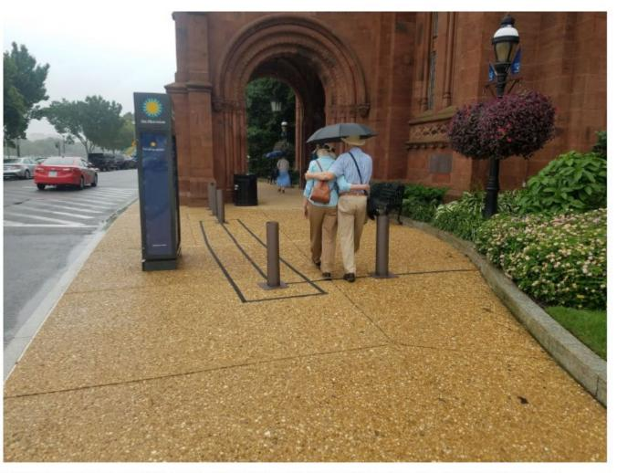
Conceptual bollard configuration at west side of porte-cochere with hardened bench massing taped-out on pavement
