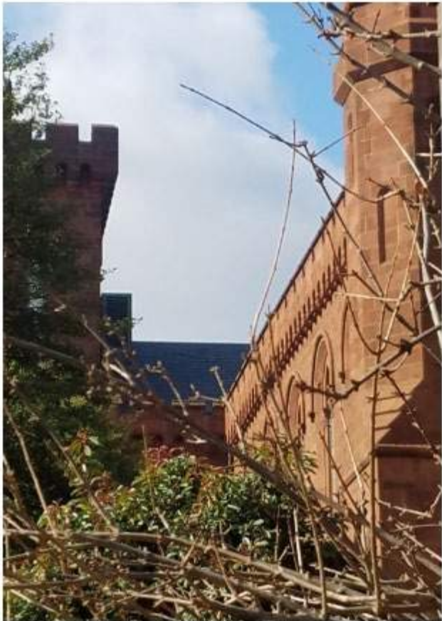
EXISTING VIEW FROM GRADE – LOOKING NW
