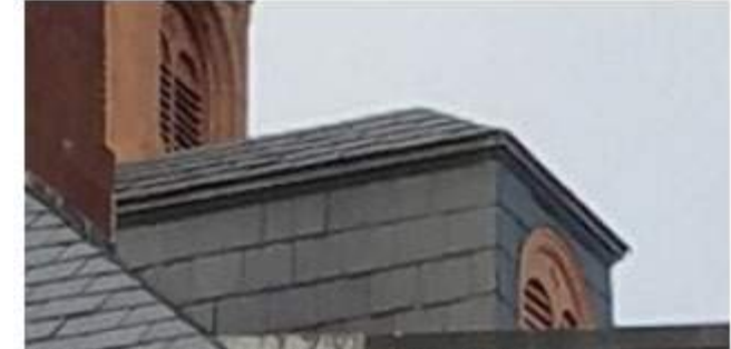
EXISTING EAST WING DORMER - SLATE
