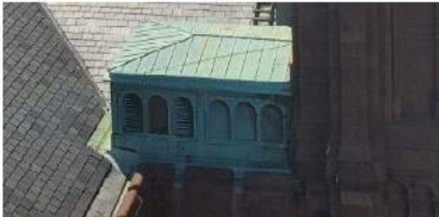
EXISTING NORTH ENTRY HYPHEN DORMER - COPPER
