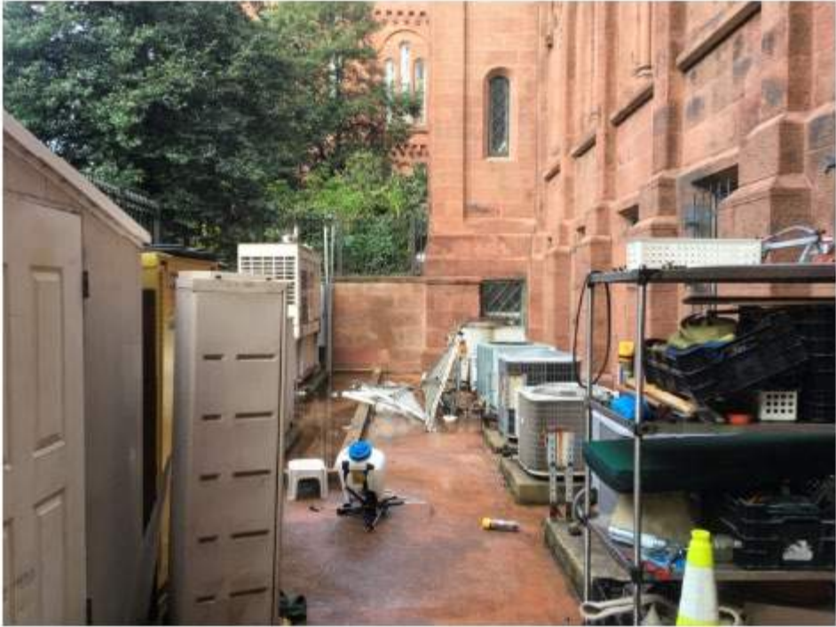
VIEW OF EXISTING MECHANICAL AREAWAY
