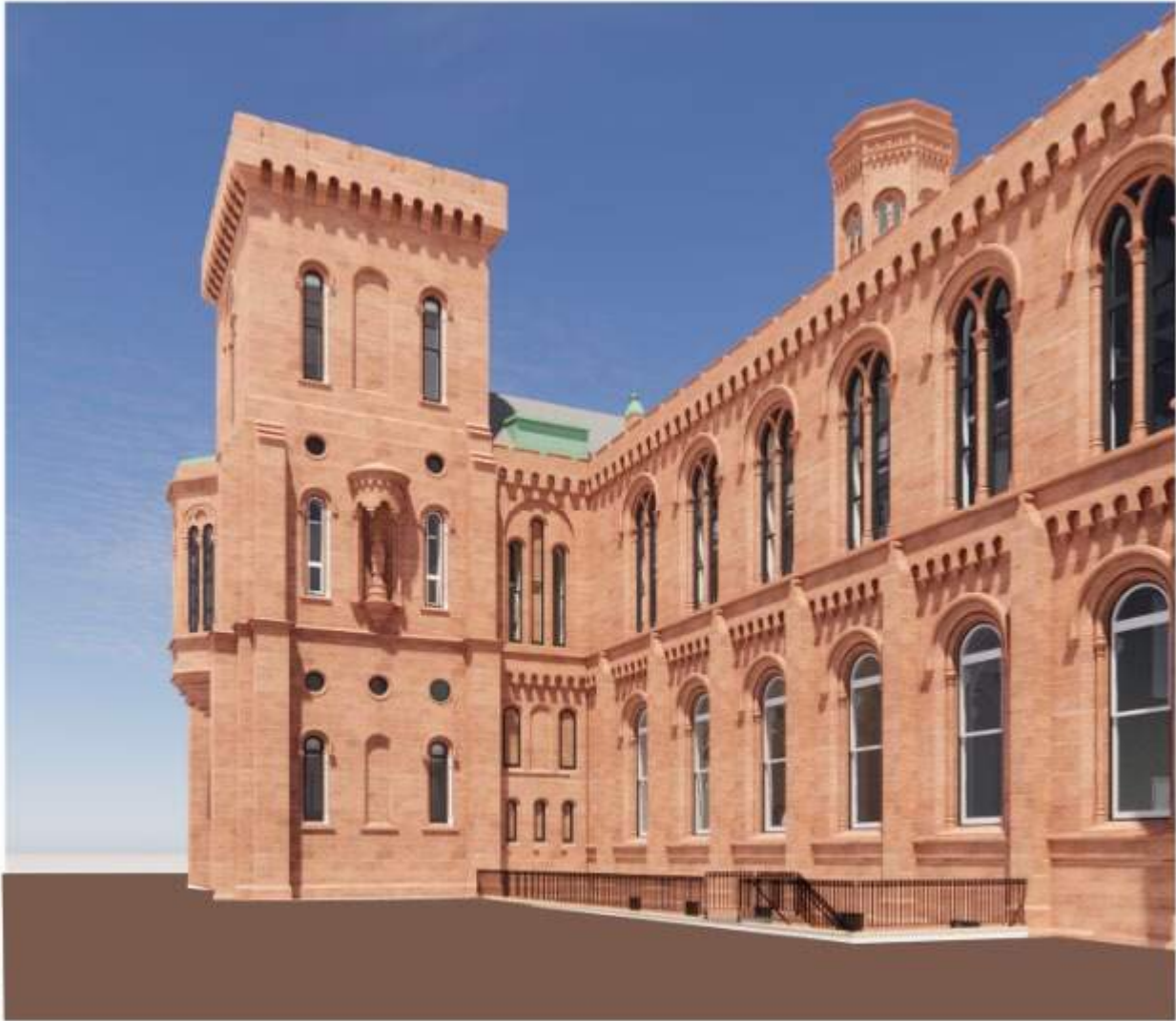
ELEVATOR OVERRUN – SLATE ROOF
