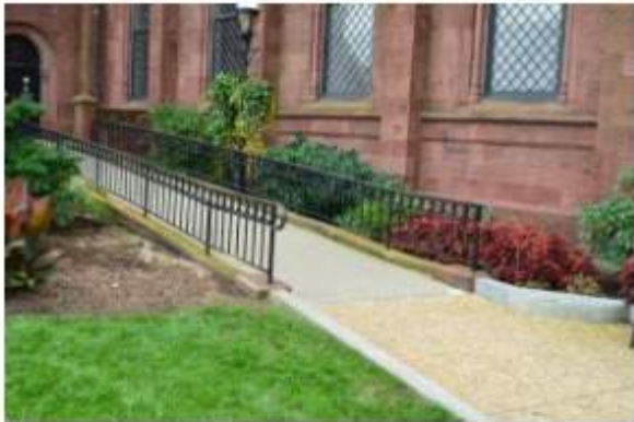
EXISTING SIB NORTH RAMP RAILING
