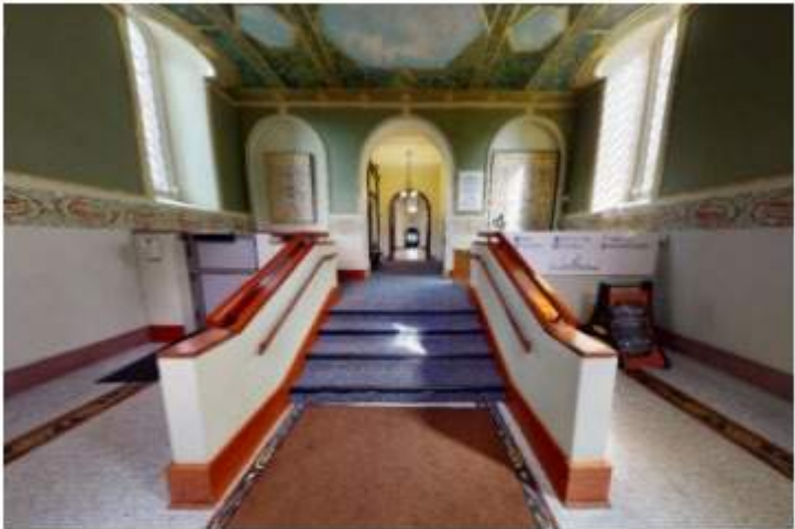
EXISTING CONDITION (looking north)
