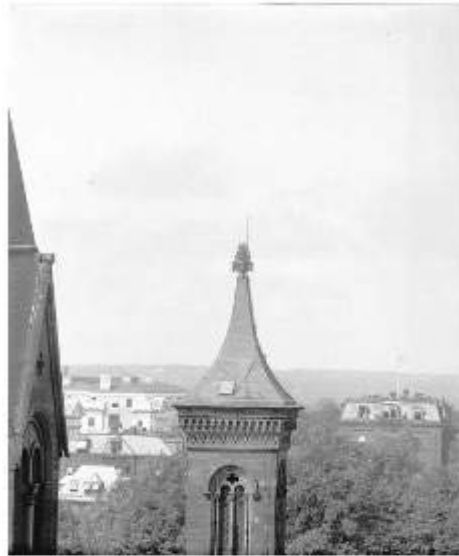
Image of the West Tower with lightning protection running up to an air terminal taken ca. 1930. Image from the Smithsonian Institution Archives.
