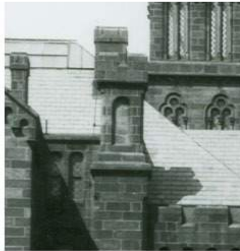
Image of the West Tower with lightning protection running up to an air terminal taken ca. 1930. Image from the Smithsonian Institution Archives.
