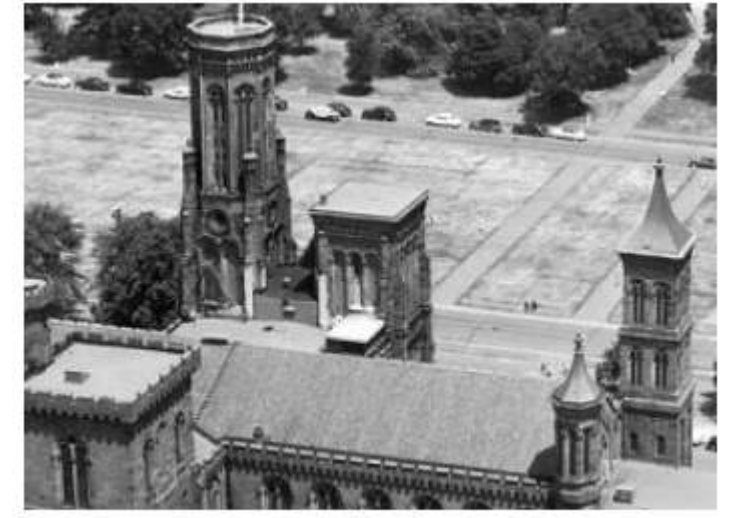
1950 North Tower and Main Roof showing established mechanical equipment. Image from the Smithsonian Archives.
