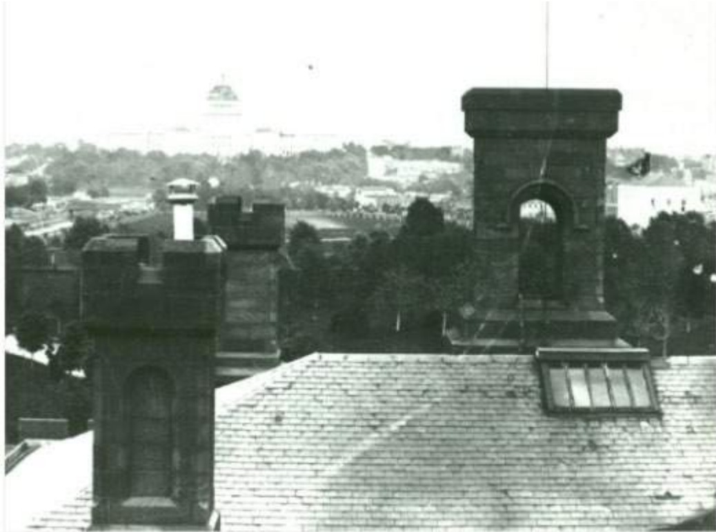
Image from 1862 of the East Wing showing an air terminal on the tower. Image from the Smithsonian Archives.
