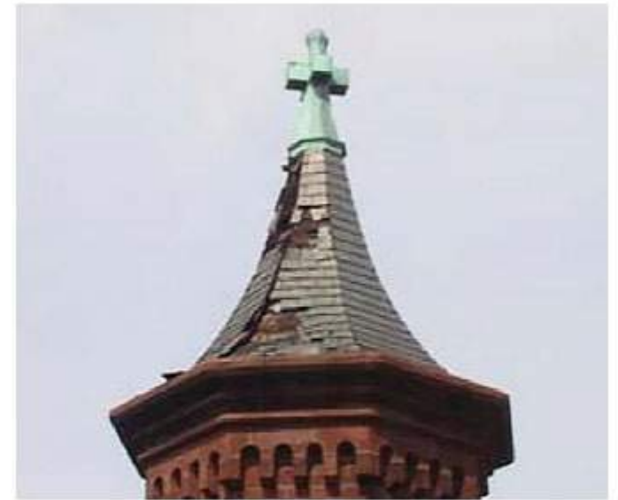
Image of the Octagon Tower damage from a lightning strike in 2005. Photo taken by Rick Stamm.
