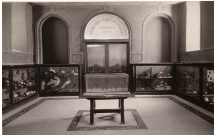
CHILDREN'S ROOM- C. 1901 (looking south)
