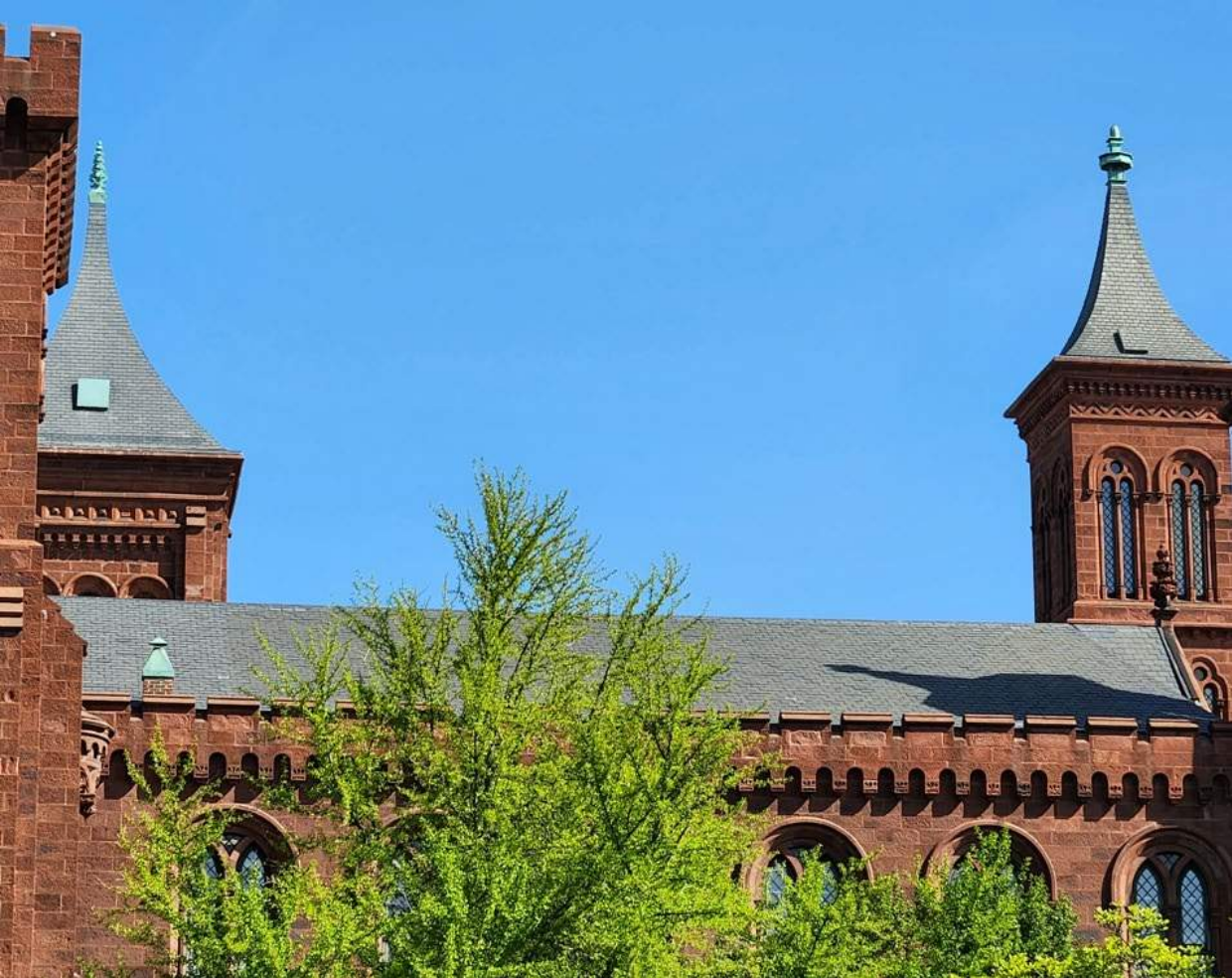
MAIN BUILDING LOOKING NORTH
