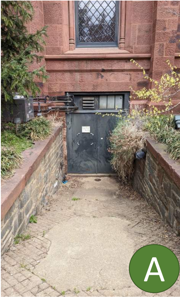
EXISTING DOOR AT SOUTHEAST OF GREAT HALL
