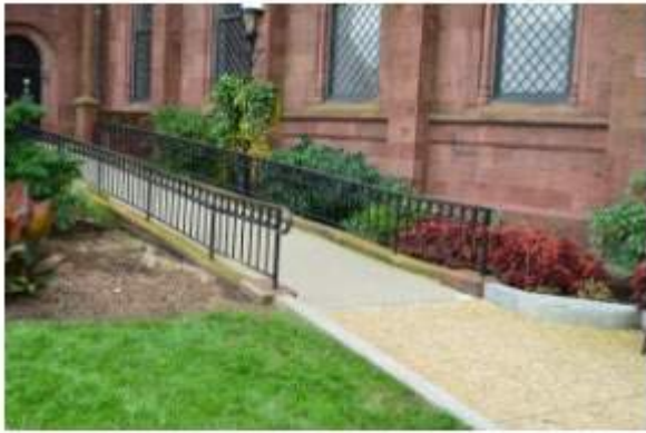
EXISTING SIB NORTH RAMP RAILING
