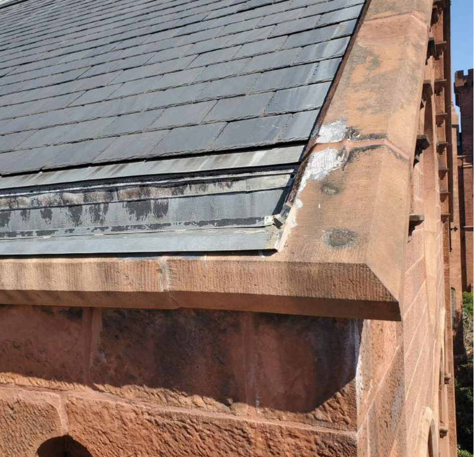
WEST WING – SOUTHWEST CORNER OF THE ROOF
