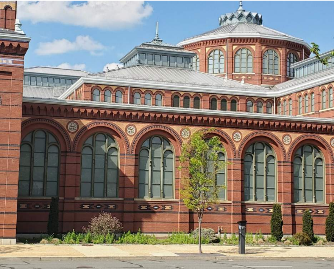
VISIBILITY OF FALL PROTECTION - FROM GROUND
