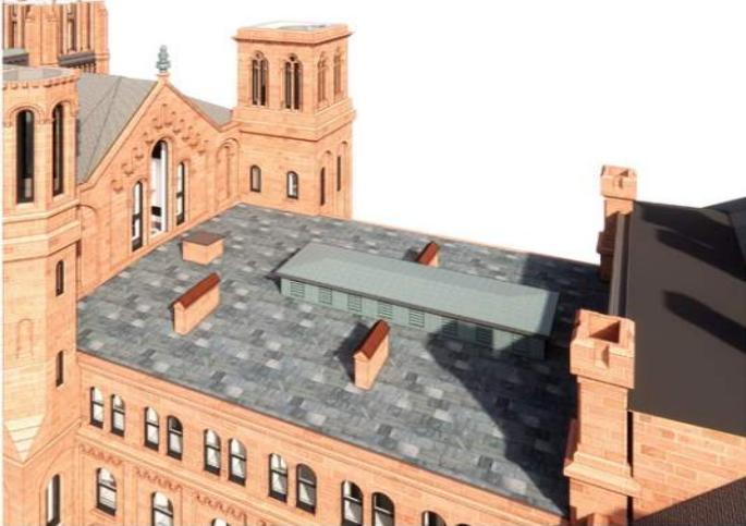
Existing Louvered Penthouse
