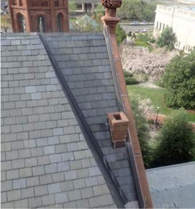
MAIN HALL – WEST END OF NORTH ELEVATION ROOF
