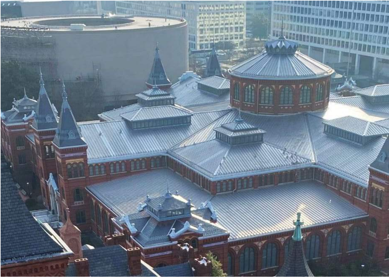
VISIBILITY OF FALL PROTECTION - BIRDSEYE
