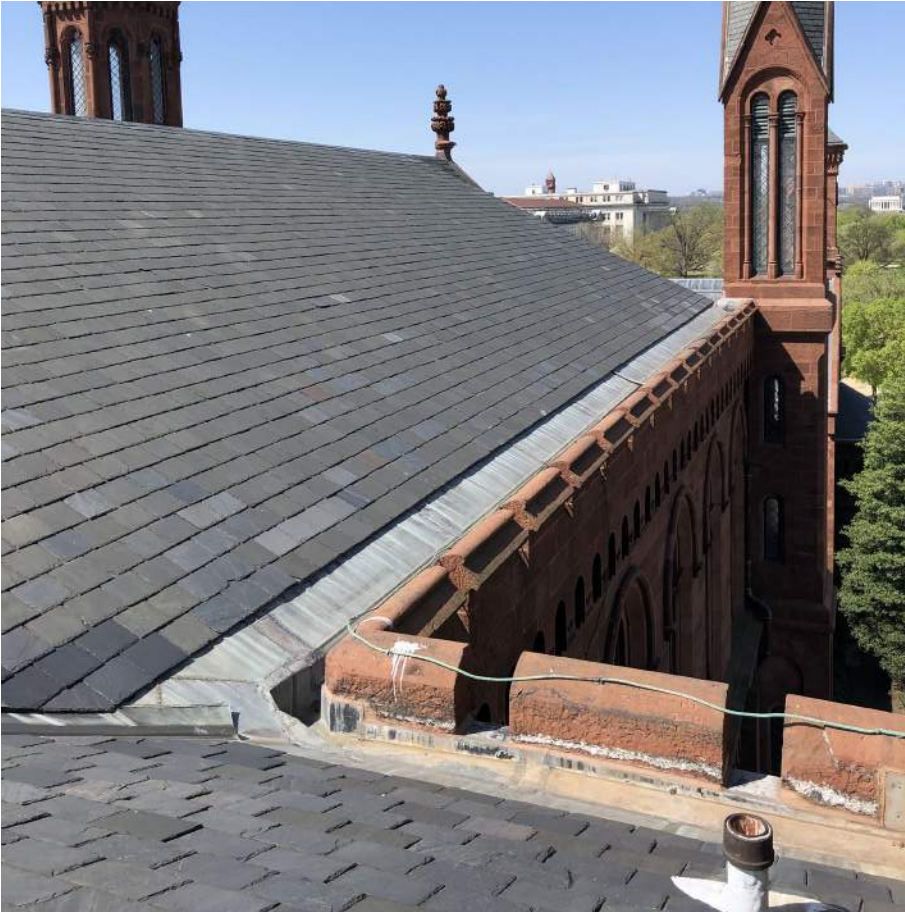
MAIN HALL – NORTH ELEVATION ROOF LOOKING WEST
