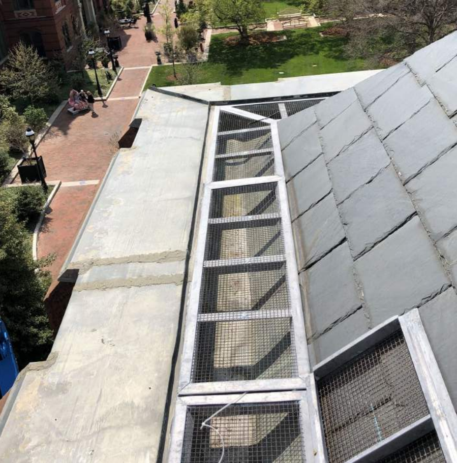
EAST WING – SOUTHEAST CORNER OF THE ROOF
