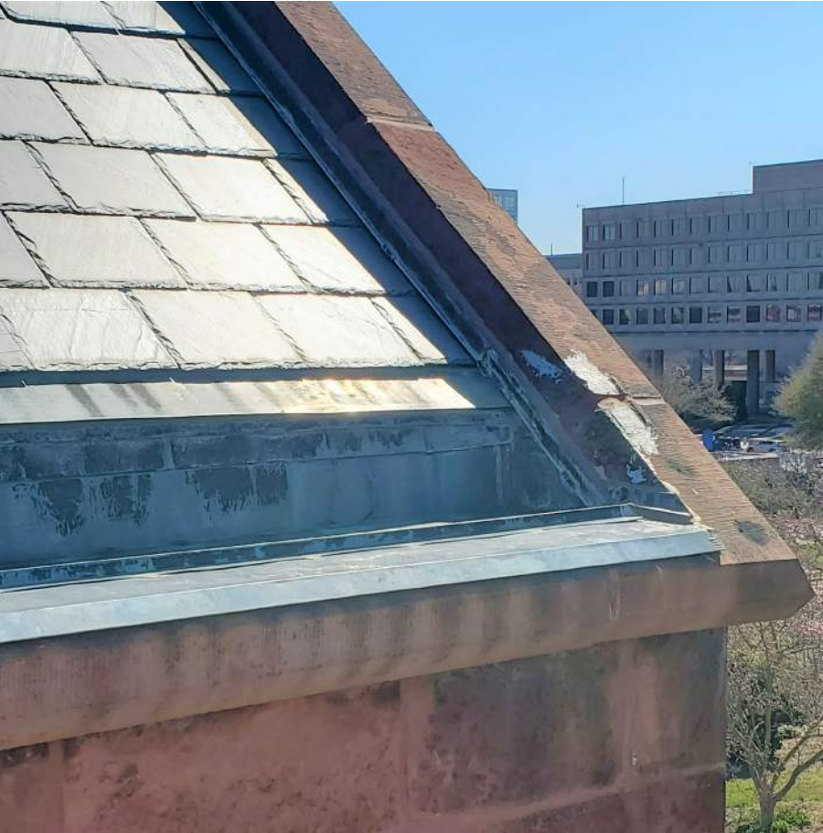
WEST WING – SOUTHWEST CORNER OF THE ROOF
