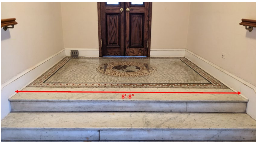
Existing upper mosaic at corridor of third level Regent's Room.
