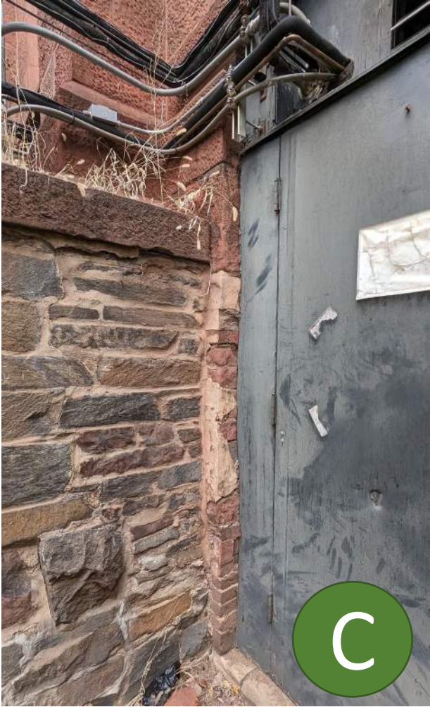
EXISTING DOOR AT SOUTHEAST OF GREAT HALL
