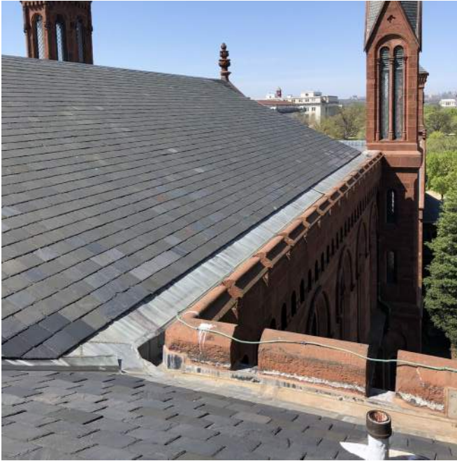
MAIN HALL ROOF EXISTING
