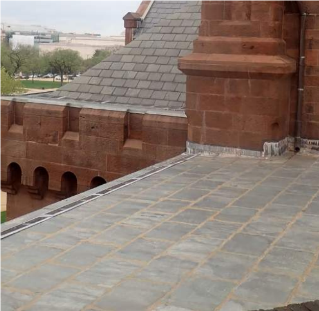
EAST RANGE & EAST WING ROOF EXISTING
