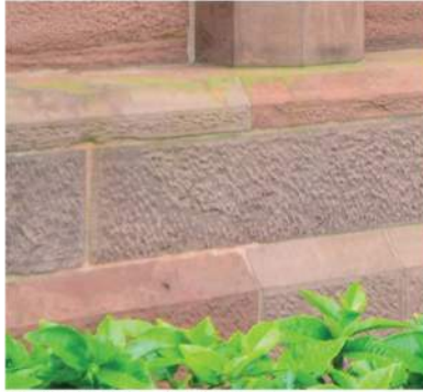
BUSH-HAMMERED SURFACE AT SIB
