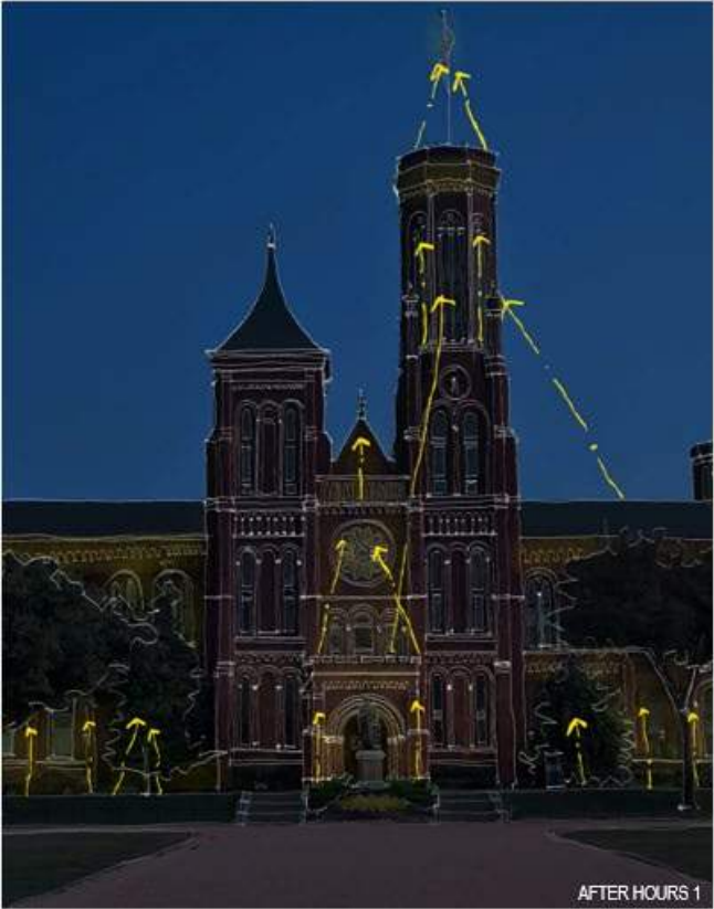
Through the control system we meet the desired dark sky considerations and preserve the building's presence in the nighttime Mall.
