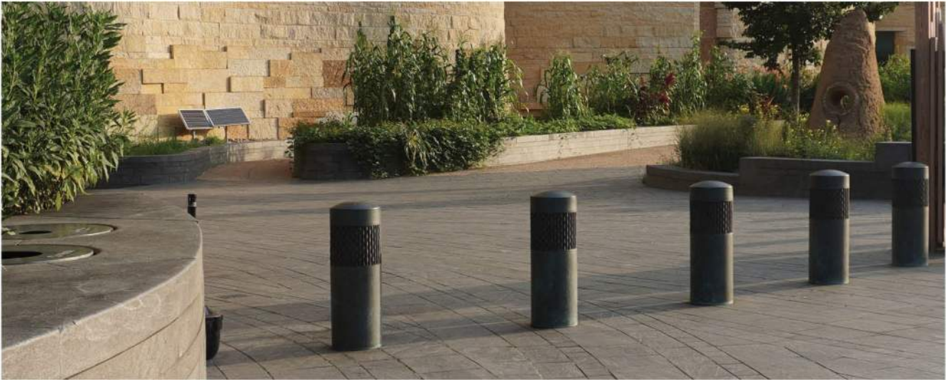
EXAMPLE OF BRONZE BOLLARD COVER (NATIONAL MUSEUM OF THE AMERICAN INDIAN), DESIGN TO BE AS SHOWN AT LEFT
