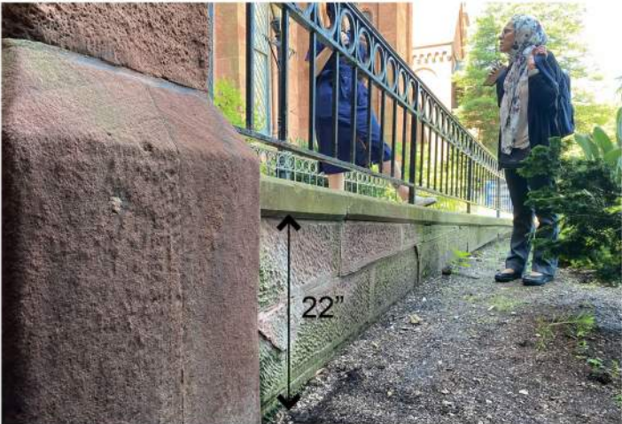
EXISTING CONDITIONS: SANDSTONE BLOCKS WITH STONE COPING
