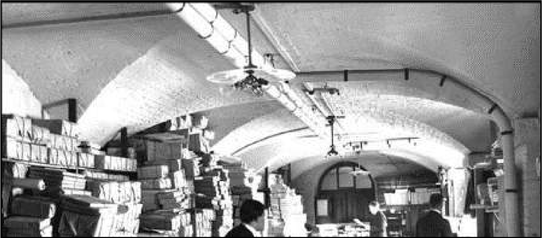
BASEMENT CEILING PAINTED WHITE
