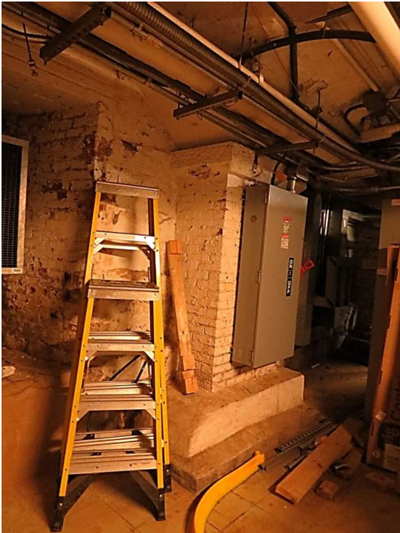
EXISTING PIER AT SOUTH ELEVATION
