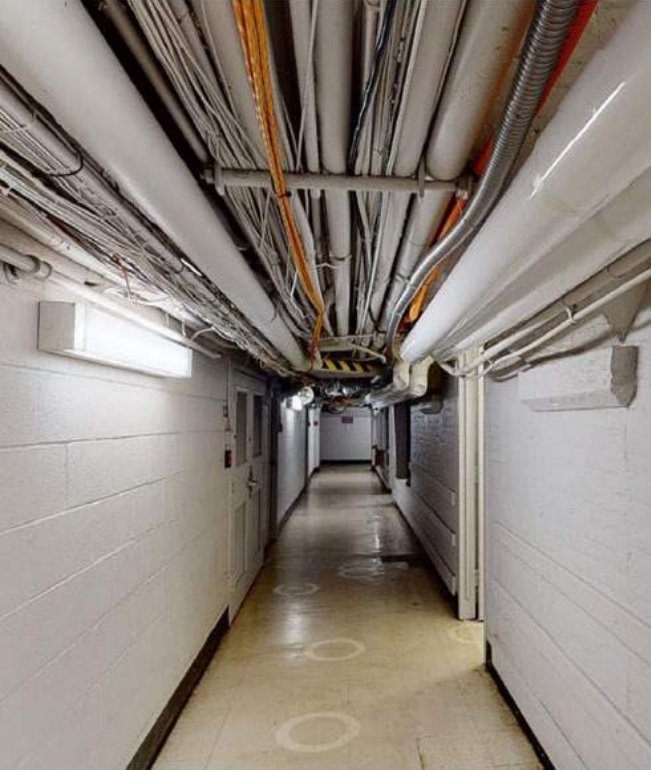
EXISTING VISIBILITY OF BASEMENT CEILING
