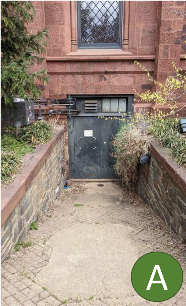
EXISTING DOOR AT SOUTHEAST OF GREAT HALL
