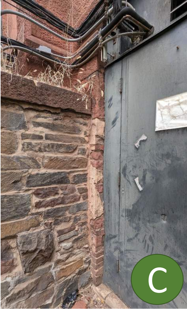
EXISTING DOOR AT SOUTHEAST OF GREAT HALL
