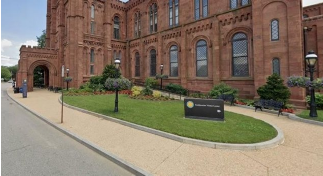
Existing west accessible ramp to the Castle's North Tower.
