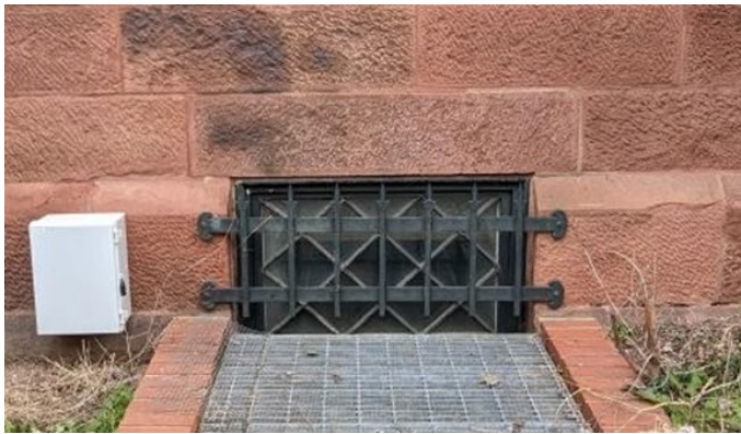
Photograph of existing basement window at the southeast side of the Main Building. Note the metal window security grille.
