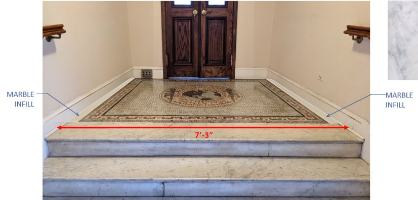
Proposed modification to the mosaics from narrowing the corridor to accommodate the elevator shafts.
