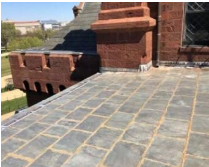
Typical conditions of slate roofing shingles.
