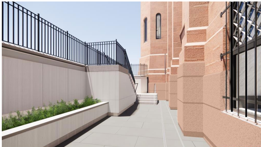
Rendering of finishes at the southwest areaway. Parging is shown on the Castle's base, gray porcelain pavers, and a neutral gray ultra-high performance concrete on the new retaining wall.
