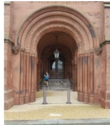
Bollard mock-up inside the porte cochere.
