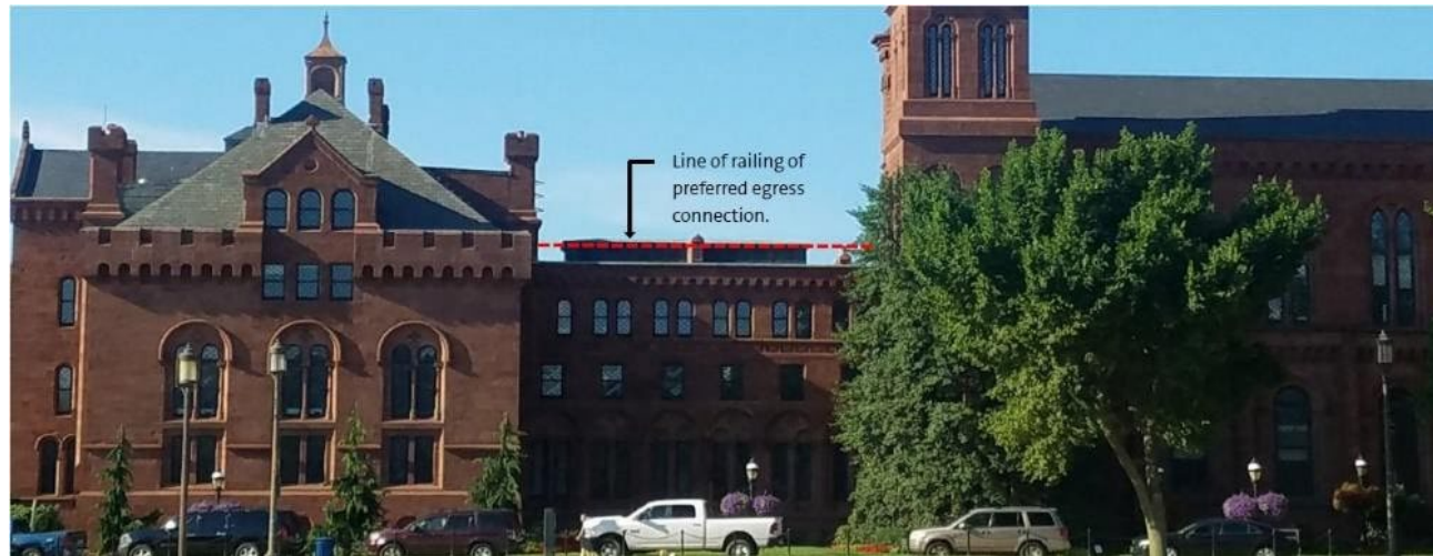
Photograph of the East Range and the visibility of the 1973 mechanical penthouse. Red dotted line indicates the height of the 42" guardrail.
