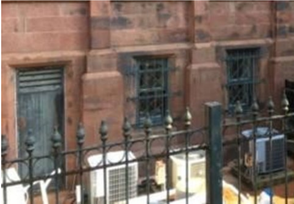
Existing egress door at the East Range south areaway.
