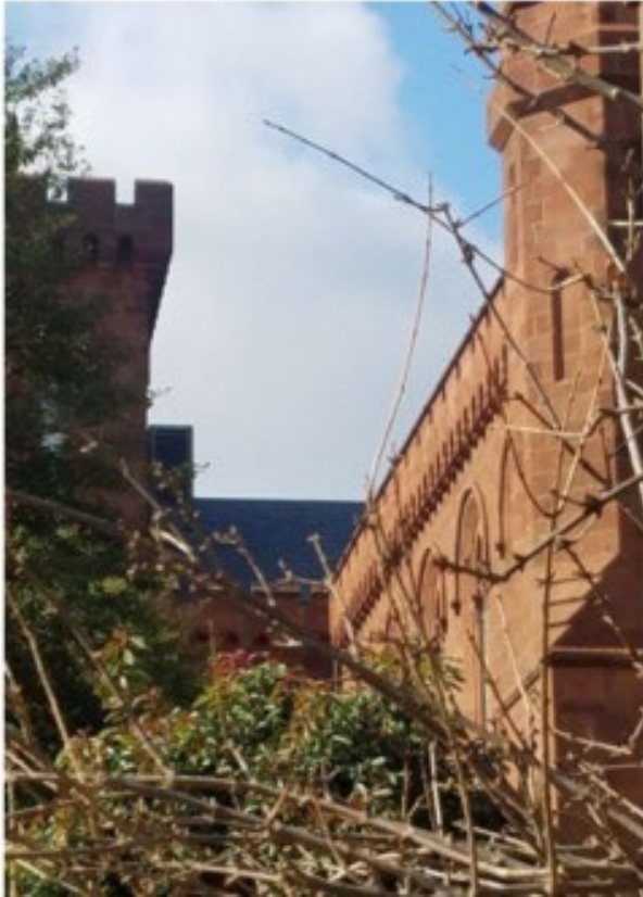
Existing view from grade looking northwest.
