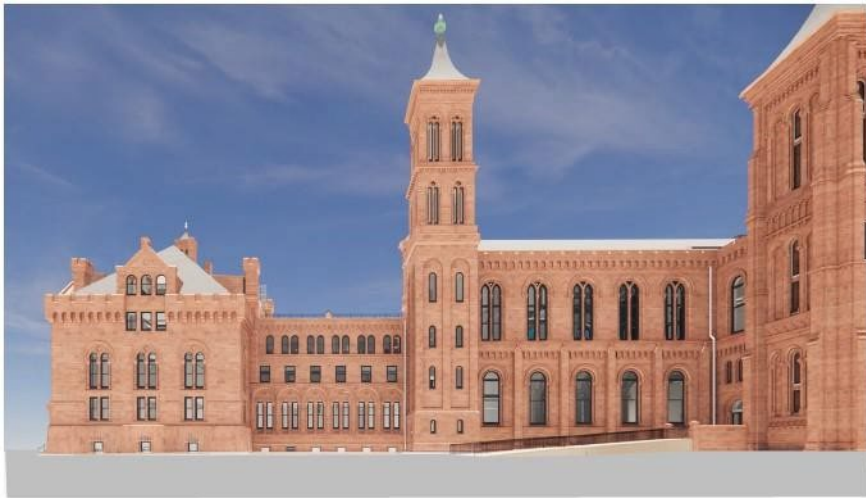
Walkway railing visibility from the middle of the National Mall.
