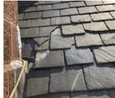
Typical conditions of slate roofing shingles.
