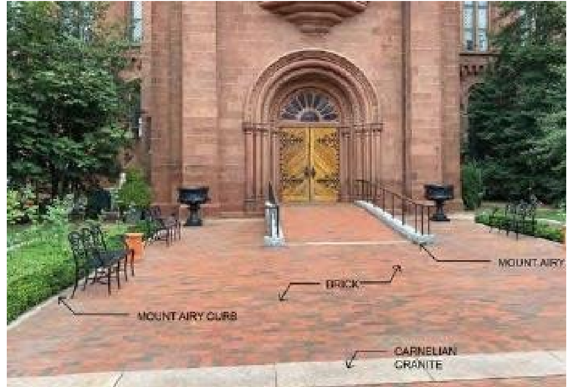
Existing South Entrance condition.
