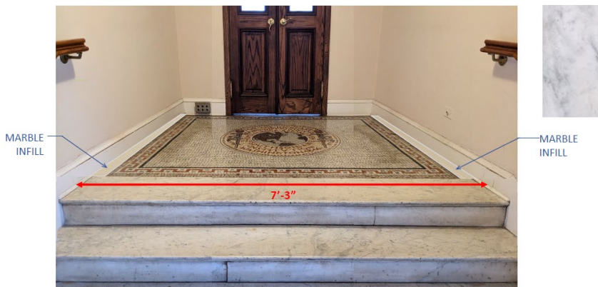
Proposed modification to the mosaics from narrowing the corridor 1'5" to accommodate the elevator shafts.
