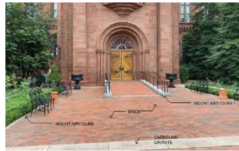
Existing South Entrance condition.
