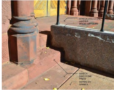
Existing ramp connection to the historic sandstone stair treads.
