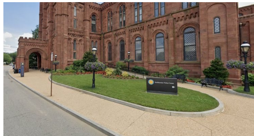
Existing west accessible ramp to the Castle's North Tower.
