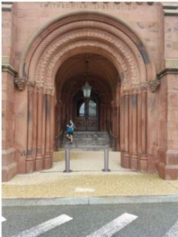
Bollard mock-up inside the porte cochere for Consulting Parties review.
