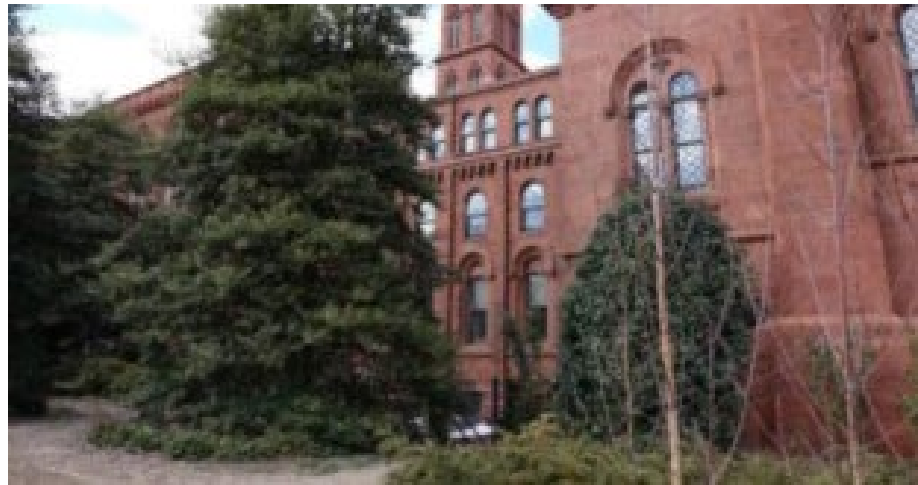
Existing southeast façade.
