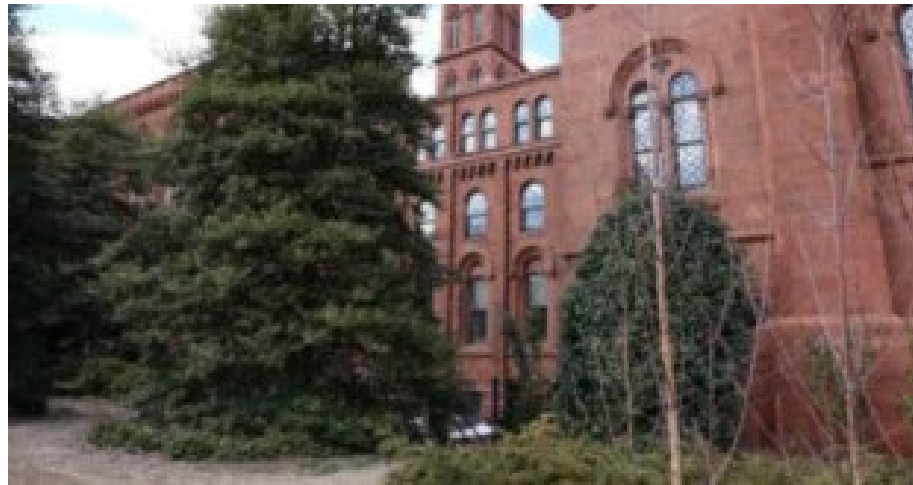
Existing southeast façade.
