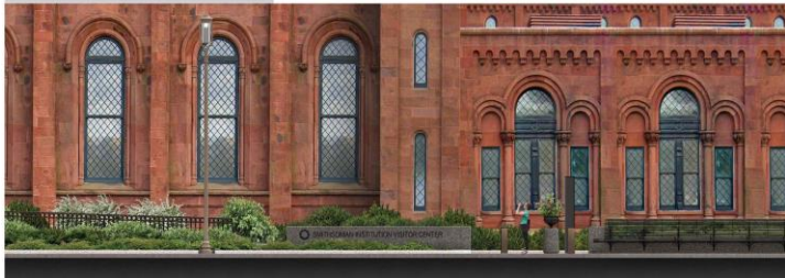
Detail rendering of perimeter security with Olympic Black granite.
