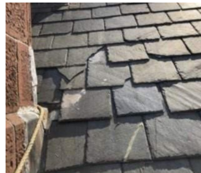
Typical conditions of slate roofing shingles.
