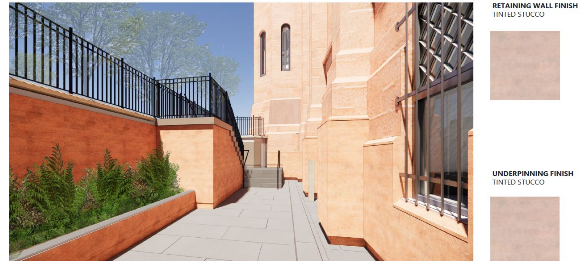
Proposed southwest areaway with red tinted stucco applied at the retaining walls and the Castle foundation wall.
