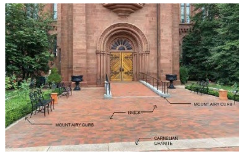
Existing South Entrance condition.
