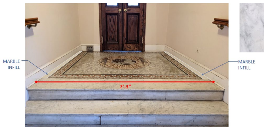
Proposed modification to the mosaics from narrowing the corridor 1'5\"/>
