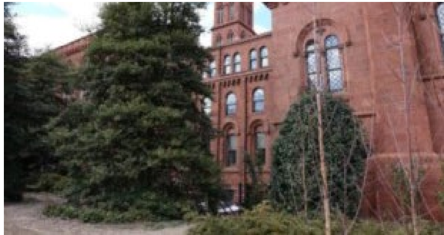
Existing southeast façade.
