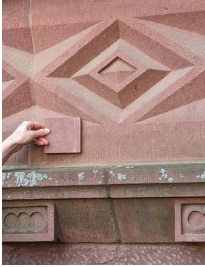
Stipulation 16.A. Use of In-Kind Replacement Materials, Exterior Masonry Repairs to Historic Fabric. St. Bees sandstone sample held against the Castle sandstone at left. Salvaged Seneca sandstone in SI storage at right.
