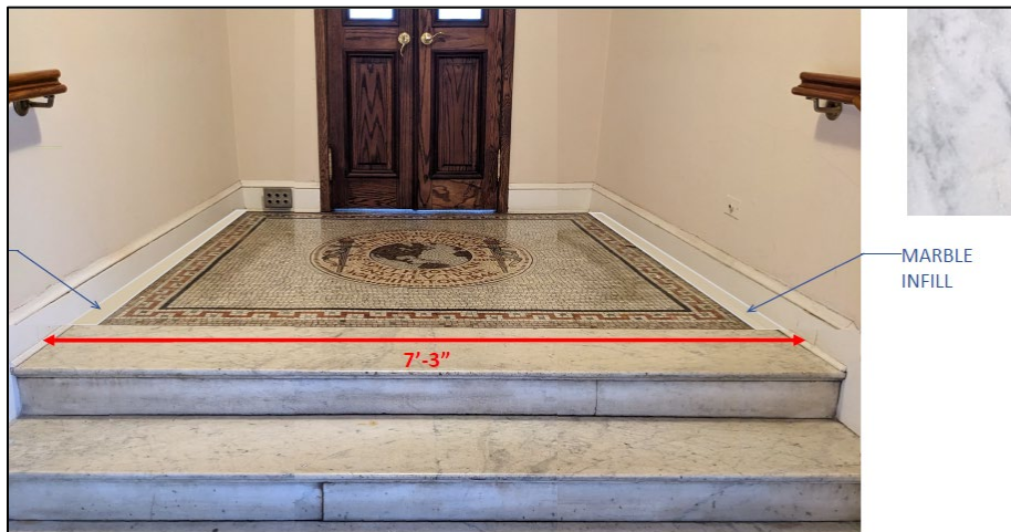
Proposed modification to the upper section of the third-floor decorative mosaic from narrowing the corridor to accommodate the elevator shafts.
