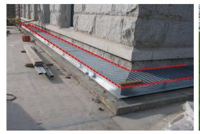
Integrated Seismic Joint Cover Examples
