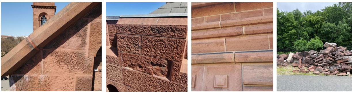
Previous Repairs on Masonry, Including Sealant in Joints and Surface-Applied Mortar Repairs
