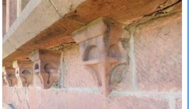
Masonry Damage Below Horizontal Projections
