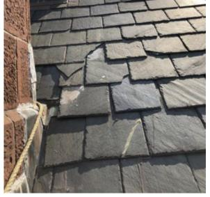
Typical Broken, Missing, or Loose Slate Shingles
