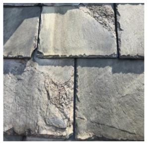
Typical Deterioration of Slate Shingles
