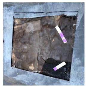
Water Below Copper Roofing, Typical
