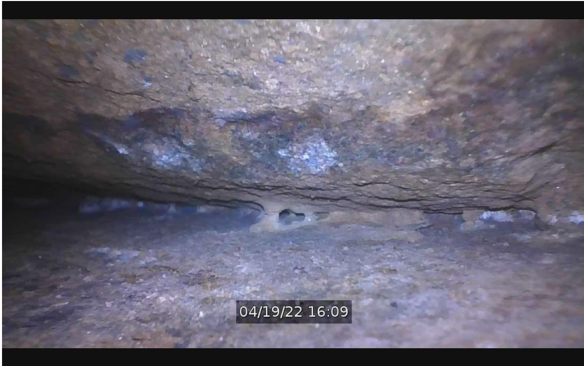
Figure 6. Videoscope image looking up inside the internal void initially suspected of being a time capsule.
