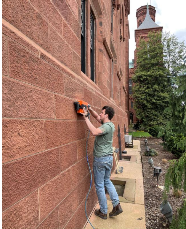
Figure 3. Typical SPR scan collected with the 900 MHz antenna at the northeast corner of the East Wing.
