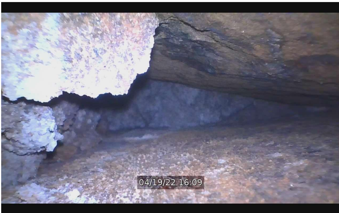
Figure 7. Videoscope image looking down inside the internal void initially suspected of being a time capsule.
