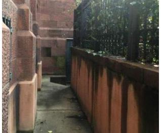
View of SW areaway – new walls were constructed of new tinted concrete while exposed foundations were parged
