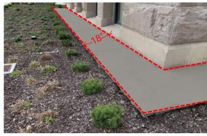
Proposed Seismic Inint Cover Detail
